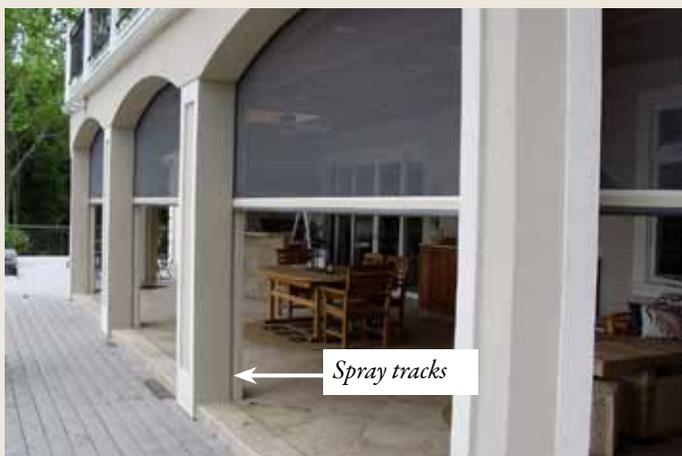
*Lubrication needs to be sprayed in the entire length of the tracks to ensure smooth operation*
