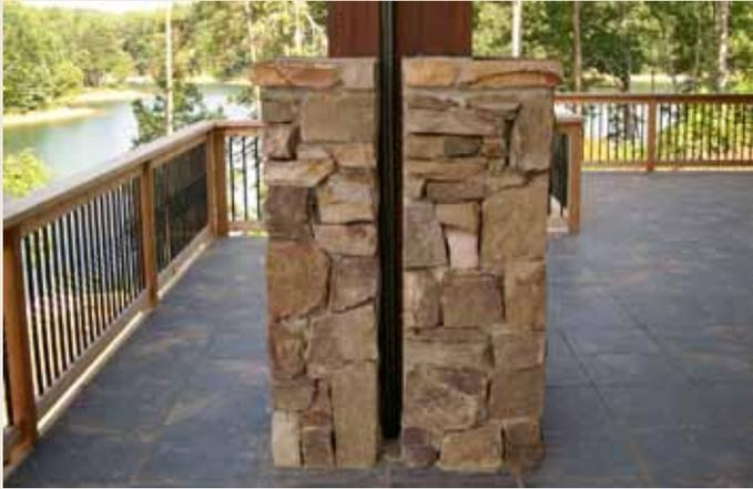
*U-channel installed within a mixed column of wood and stone*
