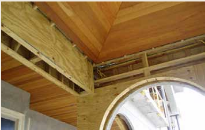
Cavity wired for installation
