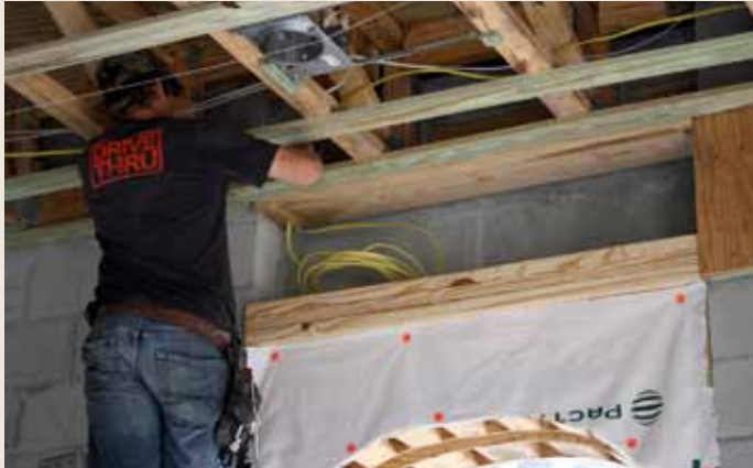
Cavity over arch being wired for 110V AC
