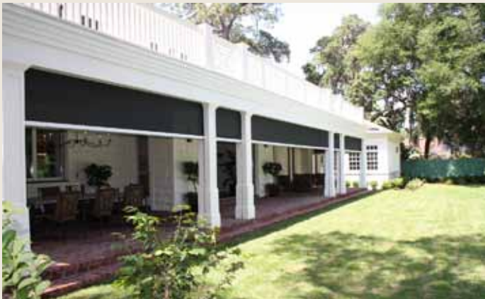
Multiple recessed Executive screens with detailed column trim
