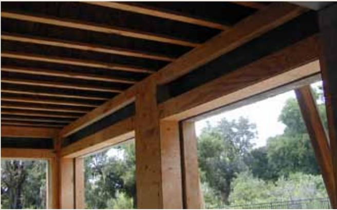
*Cavity framed in top of header opening with front access. U-channel mounted in columns surrounded by framing before stucco finish is applied.*
